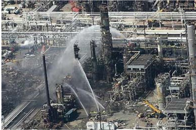
Figure 1: Fire & Explosion at Texas City Refinery 1
