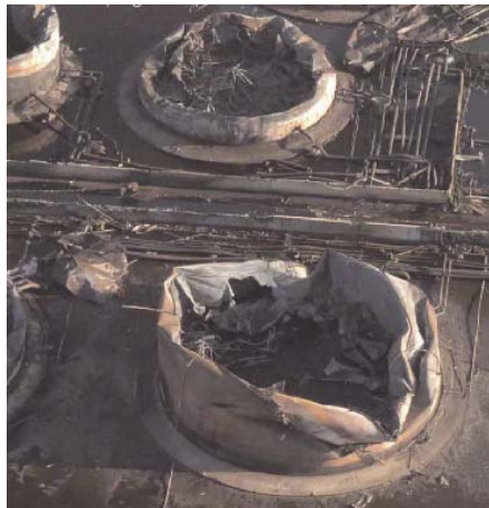
Figure 2: Aftermath of Explosion at Buncefield Oil Depot 2
